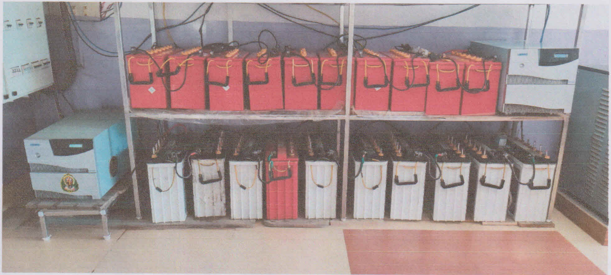
Inverter Connected with Batteries
